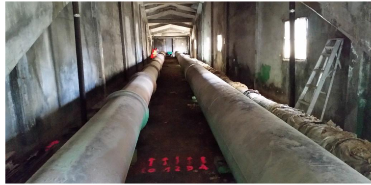
Utility investigations combine available information, field observations and targeted investigation to support project decisions.
