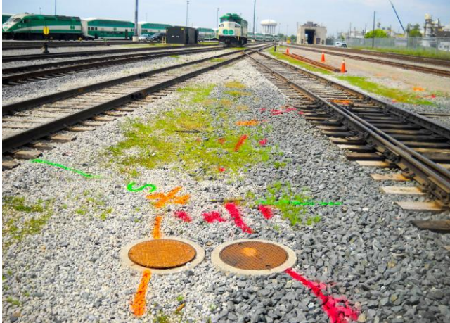
GPR and other field methods can complement electromagnetic locating where utility characteristics and site conditions warrant additional investigation.
