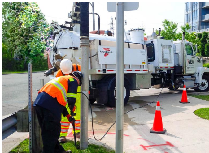
QL-A direct exposure provides precise horizontal and vertical measurement where the project decision requires that level of certainty.
