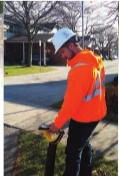
For many utilities, ground marks are considered valid for one month only, after which time they should be repainted.
